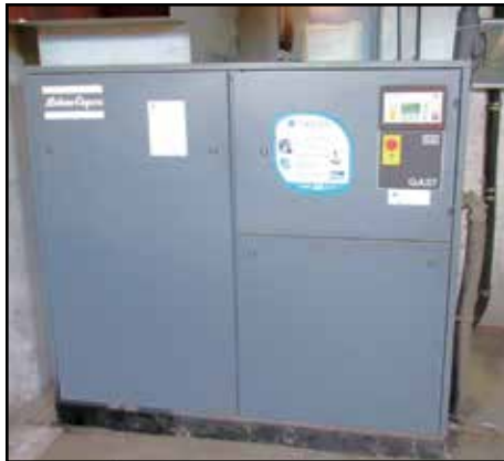
ATLAS COPCO 37KW AIR COMPRESSOR
